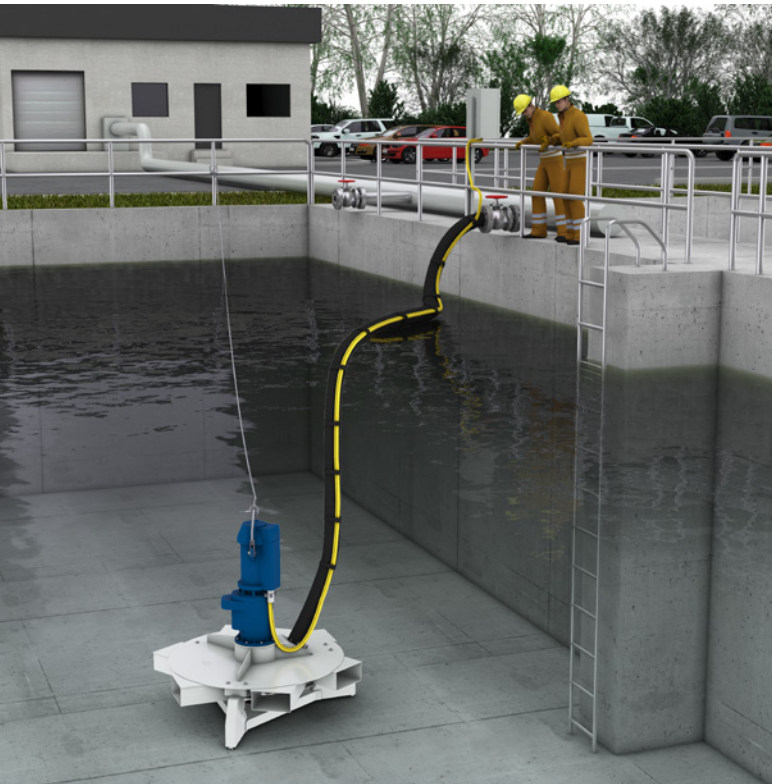
Major benefits of freestanding mechanical aerators are the ability to service the equipment while the plant is in operation and the easy addition of capacity. The picture shows an OKI aerator mixer by Sulzer fed by pressurized air.
