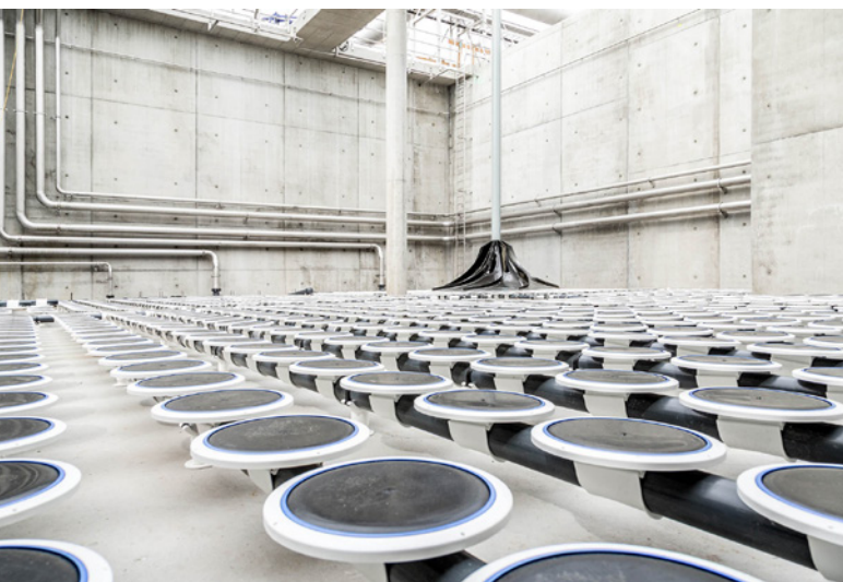
Disc diffusers are the state-of-the-art solution in aeration basins for municipal and light industrial wastewater. The PIK 300 disc diffuser from Sulzer pictured here offers durable EPDM membranes and high efficiency.
