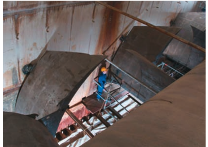
Installation of Sulzer Contour™ mixers in a large gas duct
