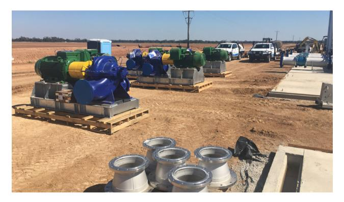
Designed from the ground up, each location had a concrete base laid before the pumps were fitted, with the building constructed afterwards. Sulzer assembled the pumps and motors on custom base units before shipping them to the sites. The simple operation of craning the pumps into position reduced the overall construction time. The first installation employs five pumps, with the other two equipped with five and six pumps respectively.
