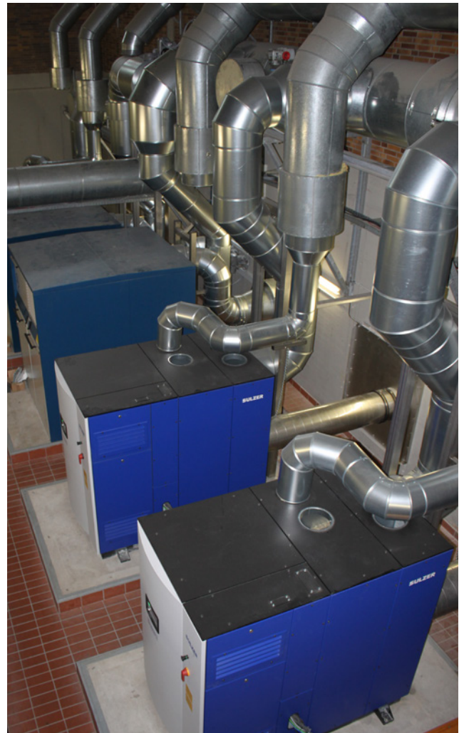
The new Sulzer HST 20 turbocompressors
