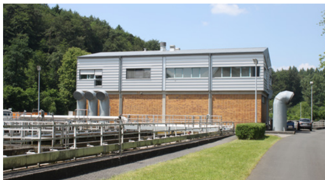
Compressor room behind the basin, intake manifolds for the aeration on the right side
