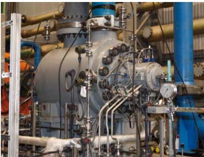
**A HPcp pump with Alloy 625 weld overlaid Carbon Steel casing for produced water injection**
