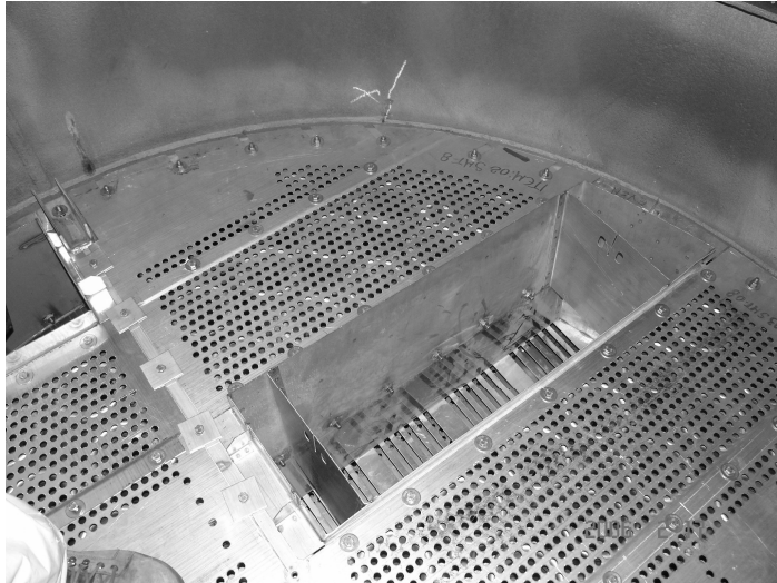
Figure 5. Picture taken during installation of ConSep tray internals for depropanizer.
