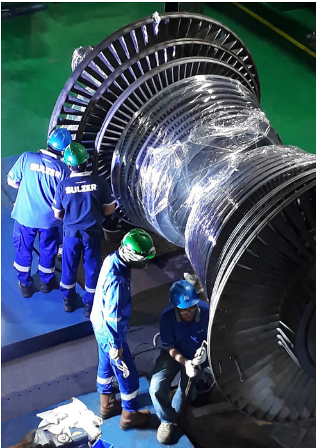
The detailed inspection revealed some of the erosion shields would need to be replaced
