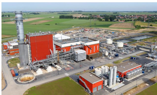
EDF Energy's combined-cycle gas turbine (CCGT) power plant at Bouchain in Northern France is one of the most energy-efficient in the world, achieving an overall efficiency level of 62.22%.
