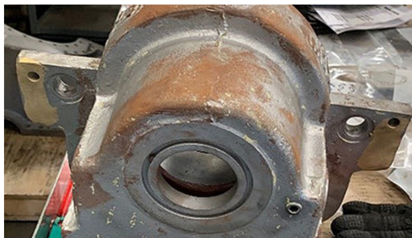
Brazed repair of the cast iron flanges
