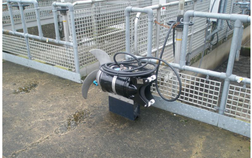
Sulzer submersible mixer type ABS XRW
