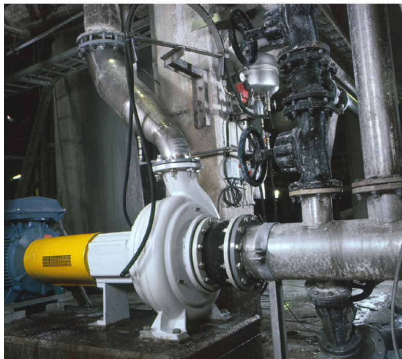
Wear-resistant end-suction pumps are designed for abrasive and erosive pumping applications.
