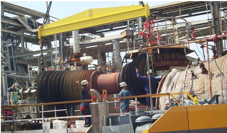
On-Site Major Overhaul of a Gas Turbine
