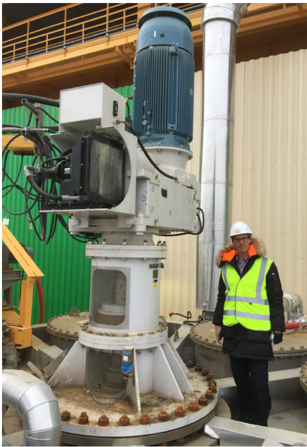
Scaba 240FVPT-Sff agitator operates smoothly at the PhosAgro Cherepovets site in Russia.
