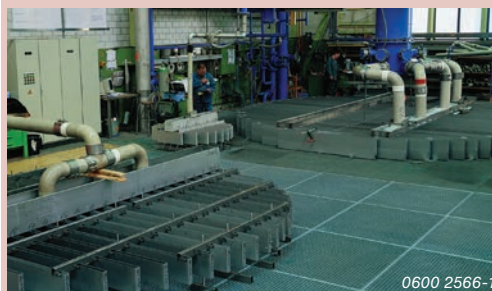
Liquid distributor test to confirm the correct operation range of each distributor
