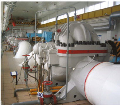
Typical pipeline pumping station
