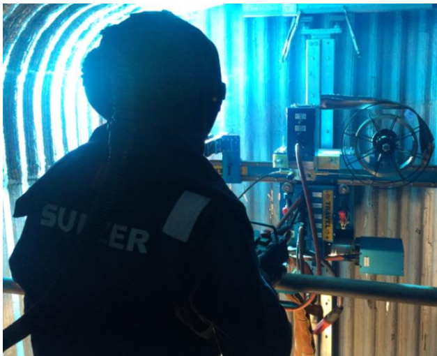
Picture 1: Automatic weld overlay
