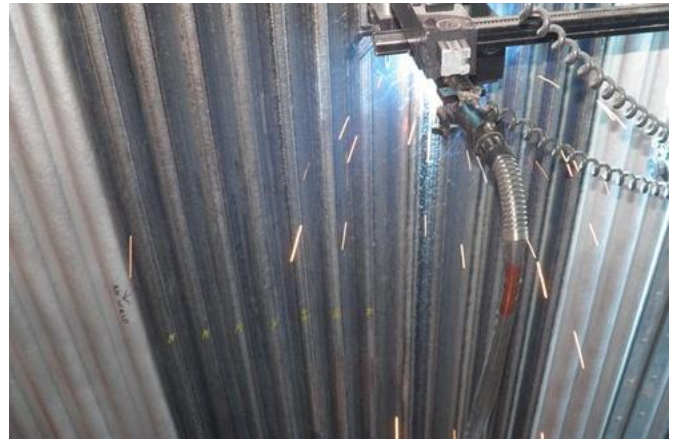
Picture 2: Onsite overlay in progress
