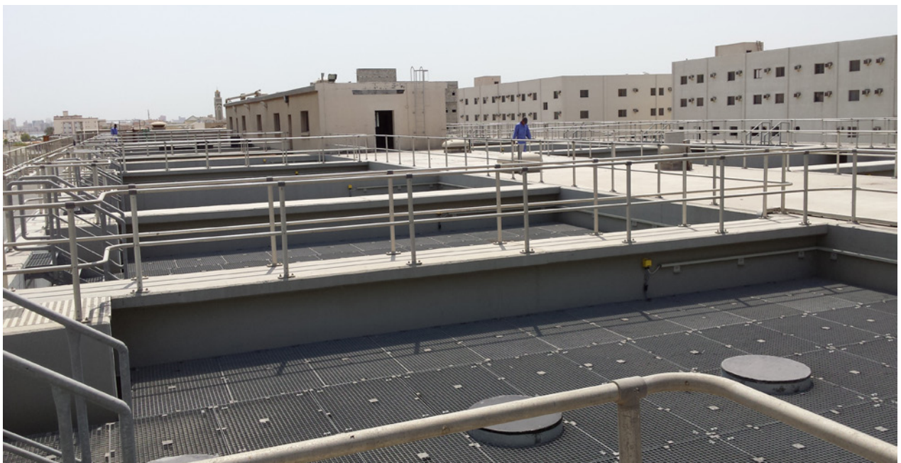
The original 20 sand filter basins were converted to DynaSand filters
