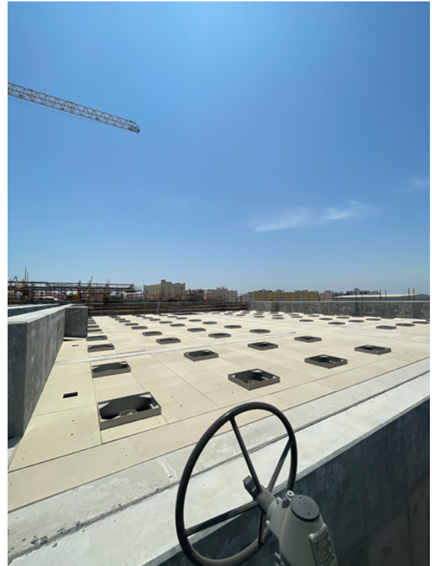
The latest expansion project used purpose-built concrete basins
