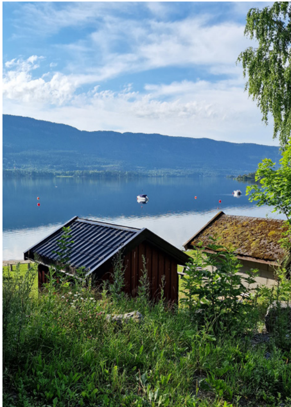
The new pumping station was designed to blend in with surrounding buildings
