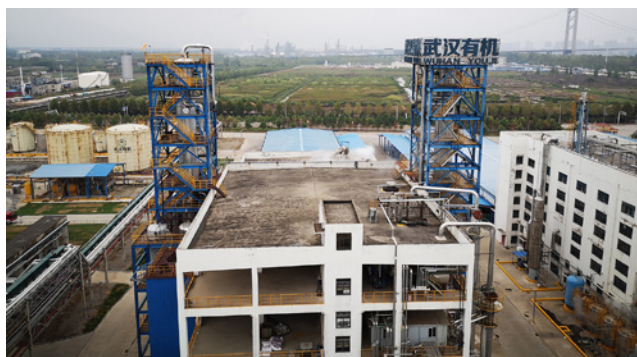
Two benzoic acid falling film crystallizers at the Wuhan Youji plant
