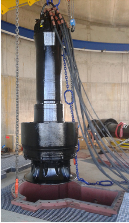
AFLX about to be lowered into riser pipe.
