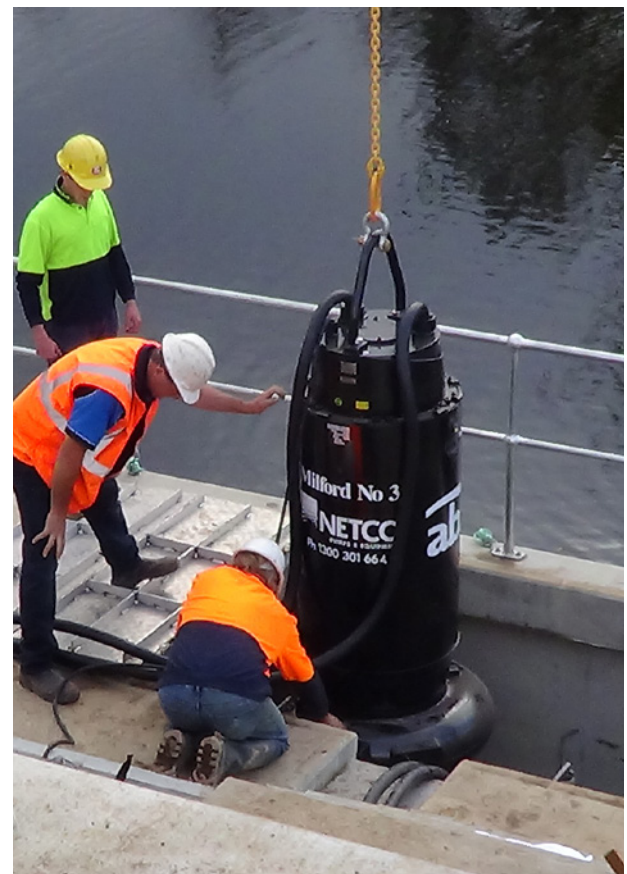
Lowering the submersible sewage pump
