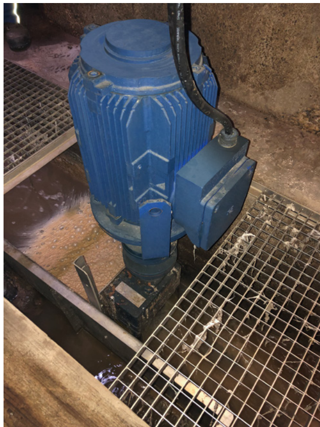
Sulzer's Muffin Monster grinder works with two shafts, fitted with sharp cutting wheels which grab, tear and cut up the material allowing the pumps to effortlessly transfer it to the next pumping station.
