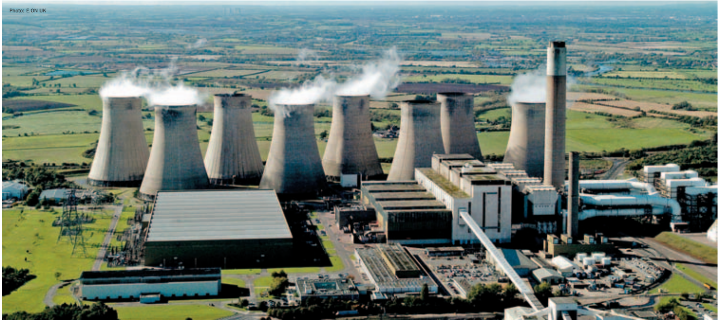
Commissioned in 1968, Radcliffe-on-Soar power station has a prominent position in the Trent valley. The plant has 4 coal-fired boilers and generates more than 2000 MW.
